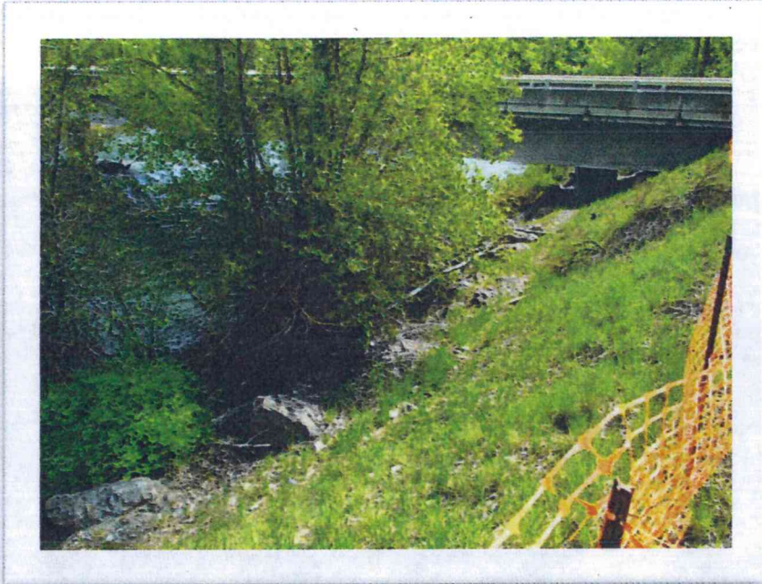
Photo 7 and 8— Shoreline conditions.
